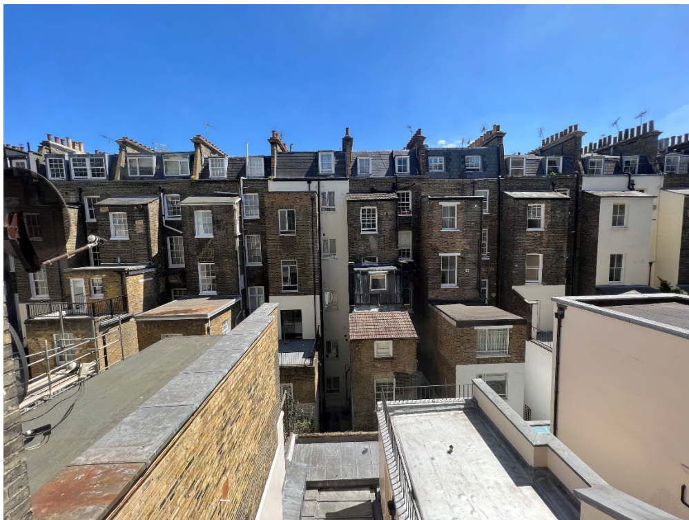
View from the rear of 54 Warwick Square
