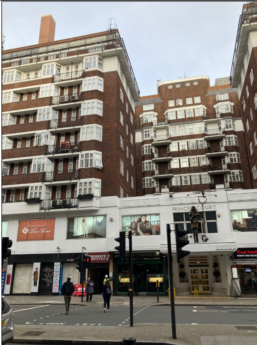
Exterior showing ground floor entrance to subject site (beneath “Rochester Big & Tall” sign).
