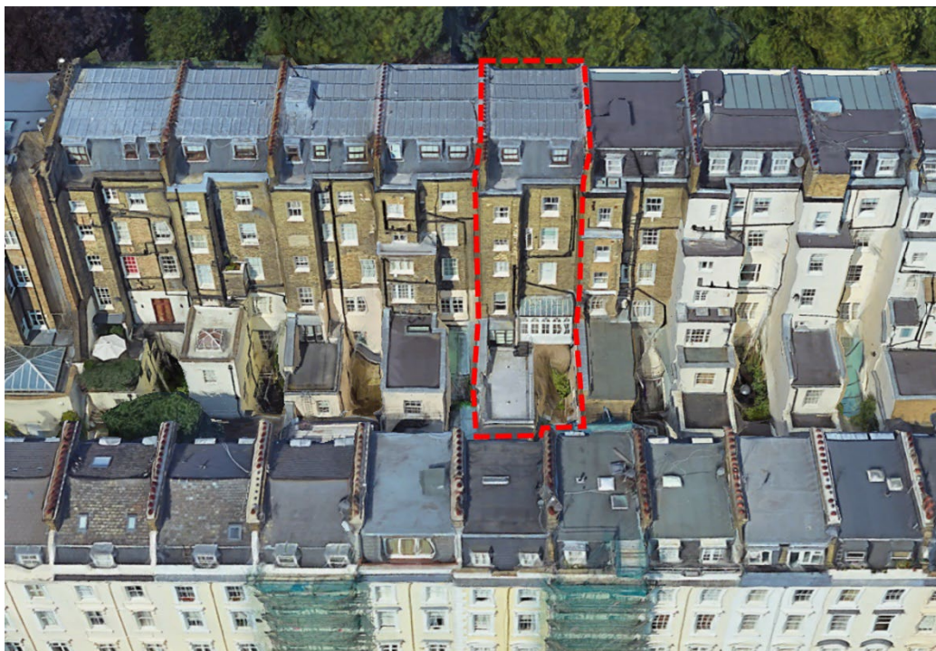
54 Warwick Square Aerial View
