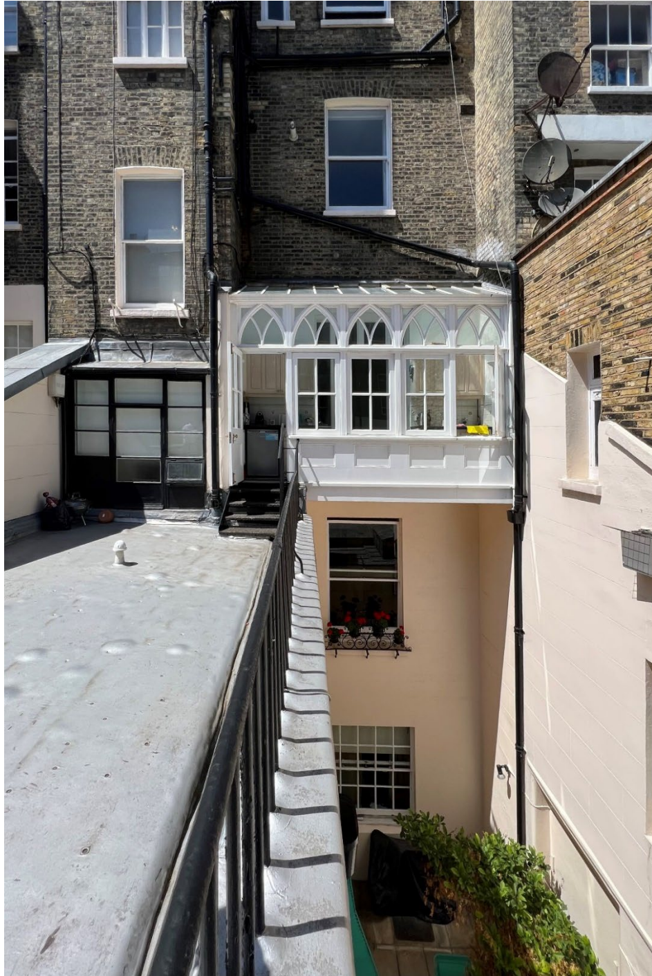
The rear elevation of 54 Warwick Square
